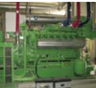
Biogas-BHKW, Reidling
